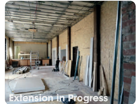
New Roof Extension
